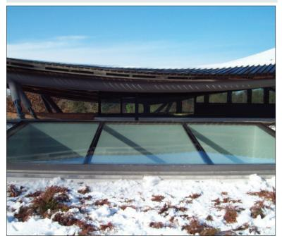
Figure 4 Typical Flushglaze installations
