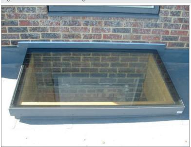
Figure 1 Wall mounted Flushglaze
